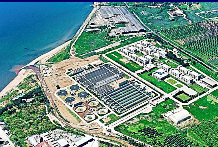
Alanya, Turkey Waste Water Treatment Plant
