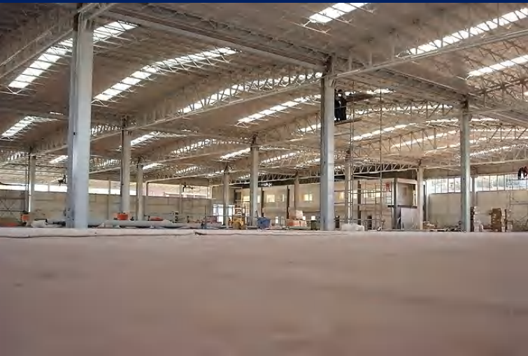
OMSAN LOGISTICS WAREHOUSE BURSA-TURKEY
