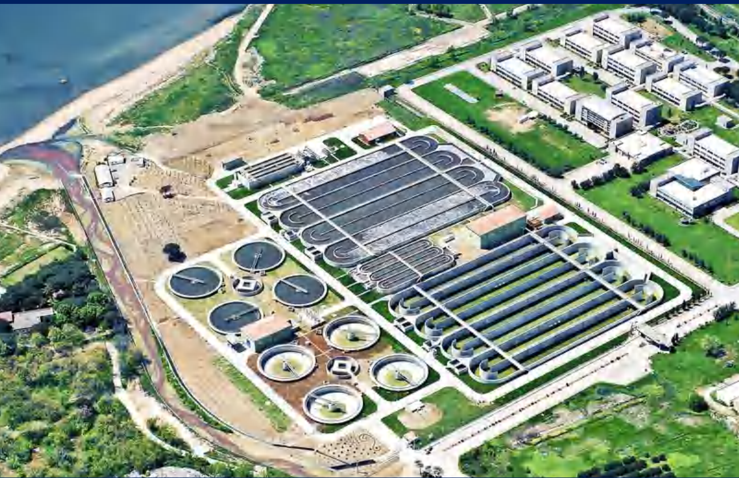
ALANYA WASTE-WATER TREATMENT PLANT
