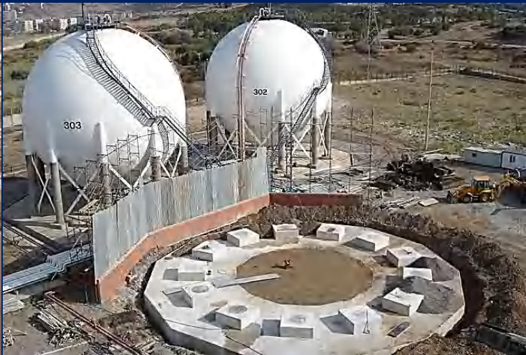
AYGAZ STORAGE TANKS & CONCRETE WORKS ALIAGA-IZMIR
