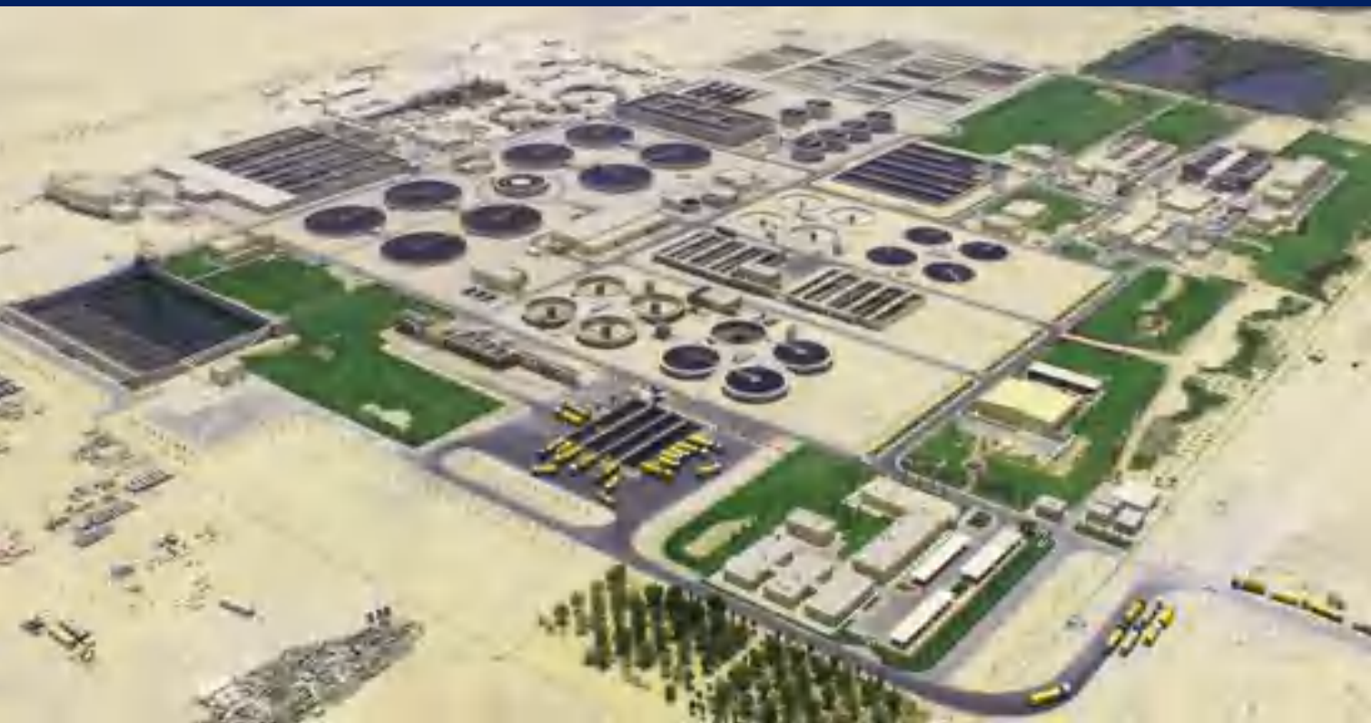
DOHA NORTH-SEWAGE TREATMENT PLANT
